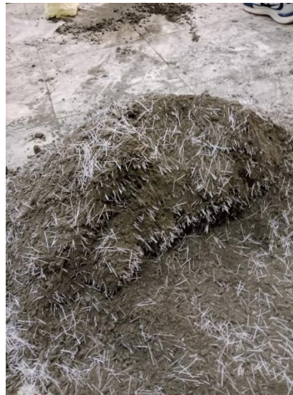
Figure 4. Dry Mixing of Material
