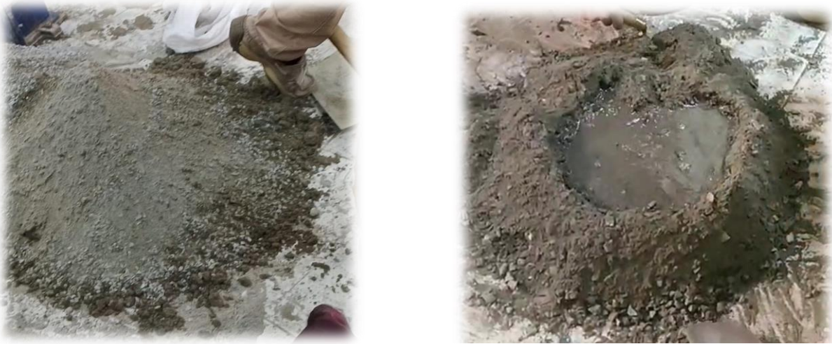
Figure 6. Mixing and casting of concrete blocks
